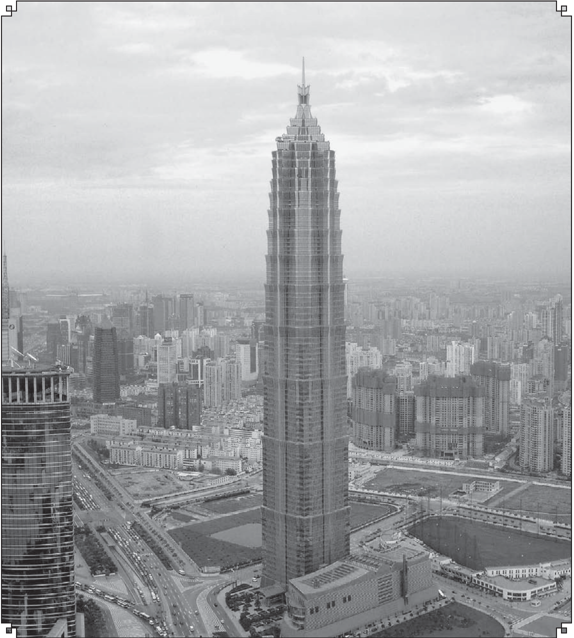
The 88-story Jin Mao Tower in the Lujiazui section of the Pudong district, Shanghai, China. © Photos.com/Jupiterimages
